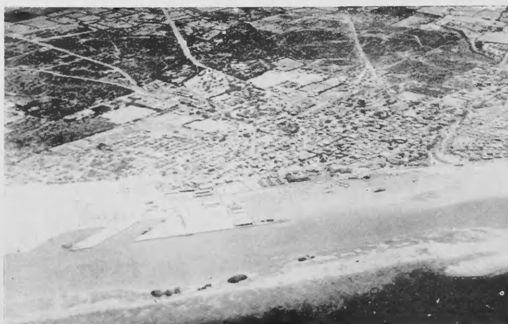
The biggest change in Oranjestad's face is the harbor development. The new ship berths and the filled land are at left in this aerial view taken late in 1949.
